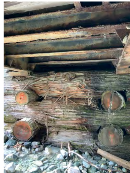
Left Bank Abutment when facing downstream
