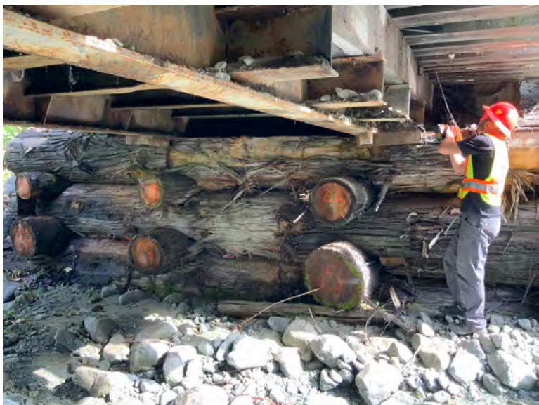
Right Bank Abutment when facing downstream
